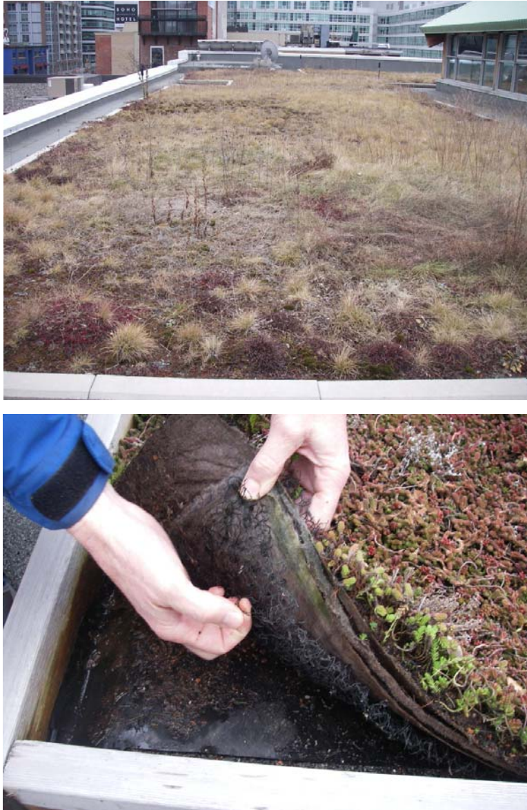
Figure 16: Extensive roof on MEC building in Toronto
