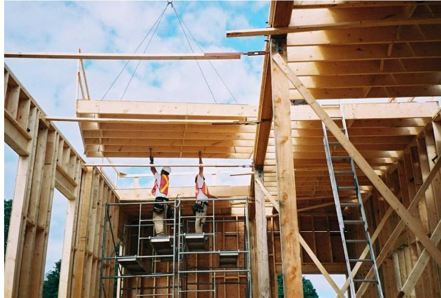
**Photo 5** BCIT Green Roof Research Facility. Prefabricated framing panel installation; built by students; installed by local contractors.
