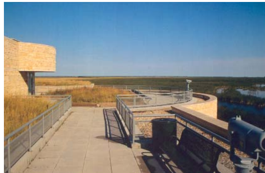
A case study of the Ducks Unlimited National Headquarters/ Oak Hammock Marsh Interpretive Centre in Winnipeg Manitoba will be presented at the workshops in Calgary and Edmonton, in December 2003.
