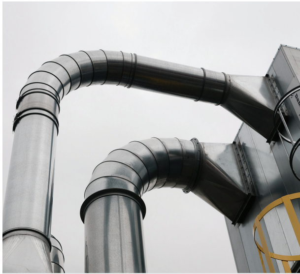
WOOD DUST EXTRACTION: DEMAND-BASED VENTILATION —SAWDUST IS EXTRACTED DIRECTLY FROM WHERE IT IS GENERATED, AND ONLY WHEN IT IS CREATED.
