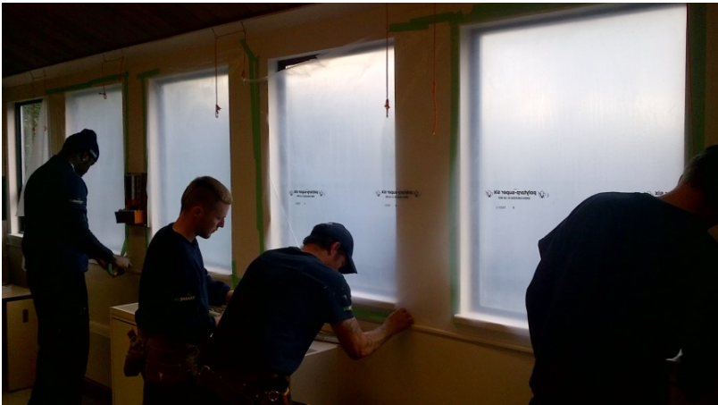
Figure 3.1 – Positioning 6 mil polyethylene before the windows removal
