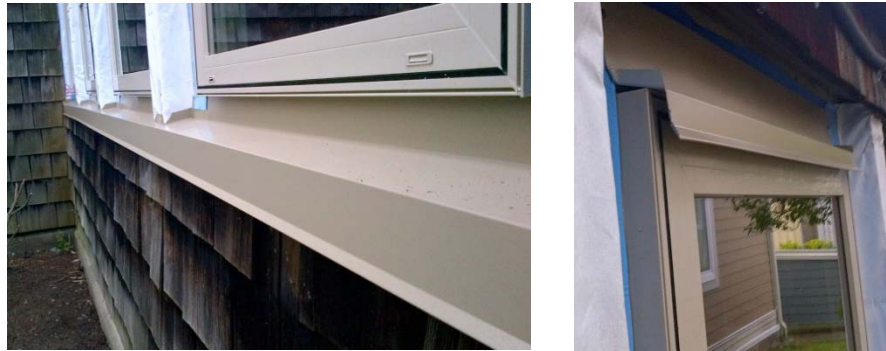
Figure 4.1 – Window flashing
