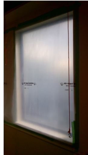
Figure 3.1 – Positioning 6 mil polyethylene before the windows removal
