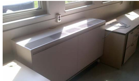
Figure 5.4 – Hydronic baseboard heaters in NE3
