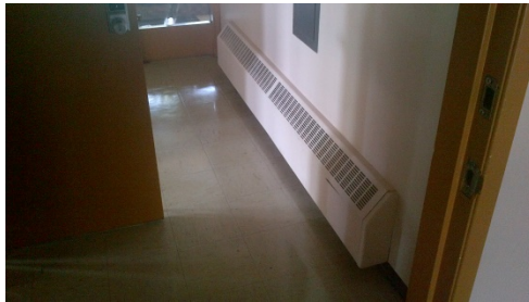
Figure 5.4 – Hydronic baseboard heaters in NE3
