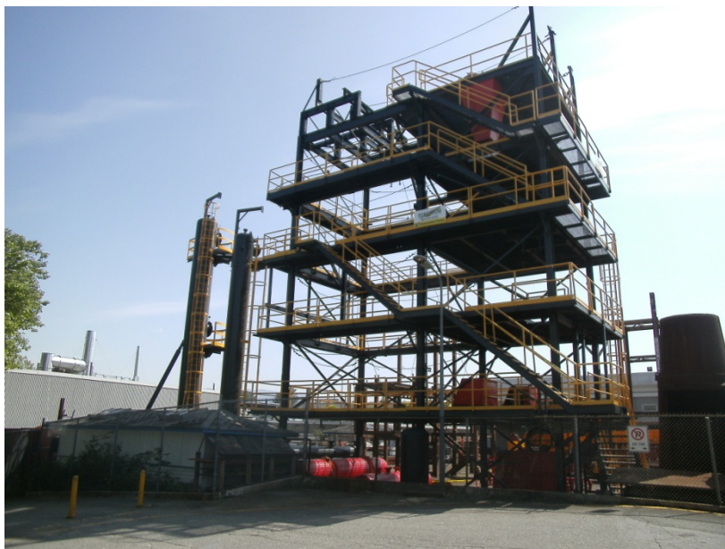
0-1: Construction at English Street
