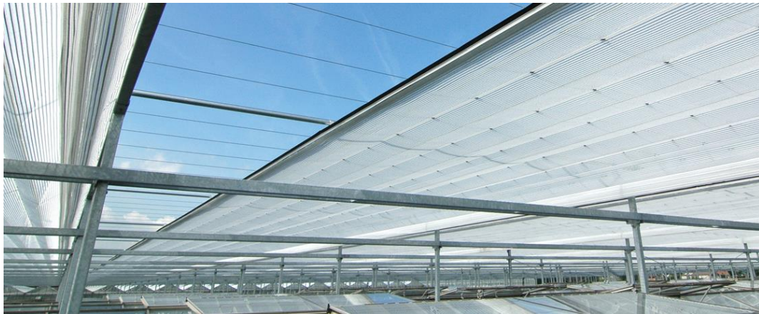
Figure 40 Skylight Shading Example: Svensson fabric shading
