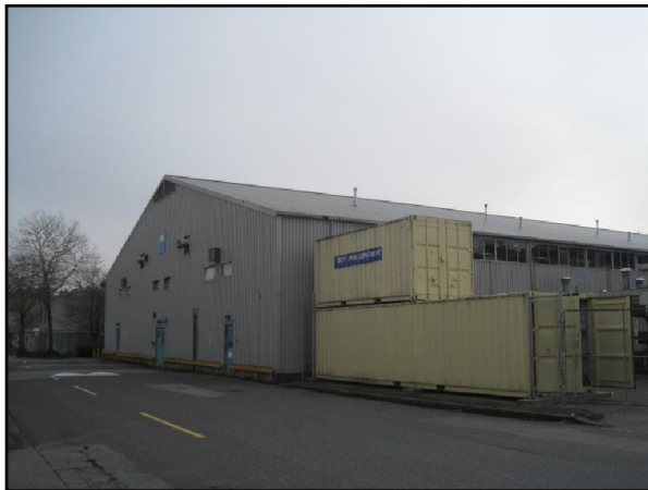
NE 6 - Plumbing & Pipefit
