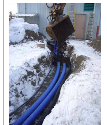
Figure 3.6 Pre-insulated flexible pipes being covered at UNBC, Prince George.
