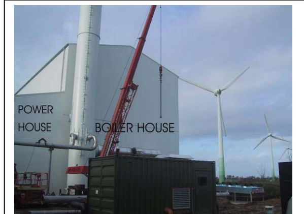
Figure 2.10 Biomass-fuelled combined heat and power plant using an Organic Rankine Cycle (ORC) technology. The plant has an electrical output of 1.6 MW.
