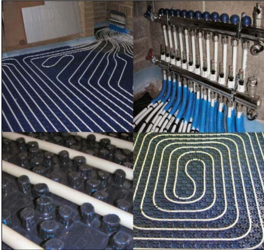
Figure 4.4 In-floor radiant heating using PEX pipes on top of an insulating vapour barrier. Heating with renewable or decentralized energy requires low-temperature consumers such as hydronic in-floor heaters to be effective. Hydronic floor heating operates at supply temperatures of 35°C. When used for education purposes, part of the floor might be covered by glass rather than concrete. Source: http://www.radiant-floor-heating.com/
