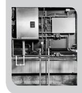
The Piping Department students installed a high efficiency condensing boiler system operating with efficiencies at up to 98%.
