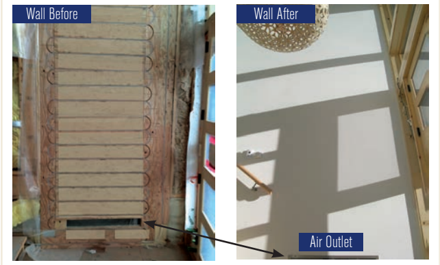
PHOTO 4 Radiant walls fabricated with drywall on PEX-a in plywood tracking on aluminum heat transfer plates on insulation, were added to the bathroom, foyer and loft areas for supplemental heat and to help reduce down drafts and reduce radiant asymmetry. Shown north wall of foyer, note air outlet for additional supplemental heat.
