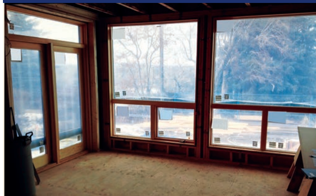
PHOTO 2 Looking out through living room windows from kitchen/dining area.
