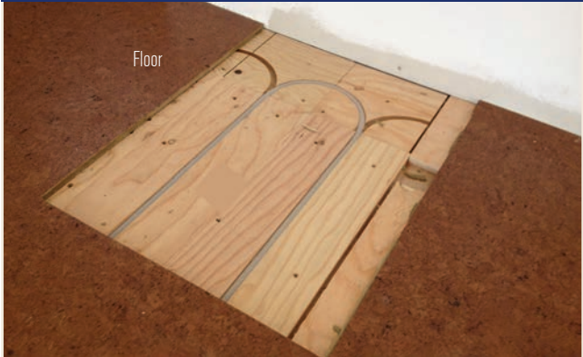
PHOTO 4 Radiant walls fabricated with drywall on PEX-a in plywood tracking on aluminum heat transfer plates on insulation, were added to the bathroom, foyer and loft areas for supplemental heat and to help reduce down drafts and reduce radiant asymmetry. Shown north wall of foyer, note air outlet for additional supplemental heat.
