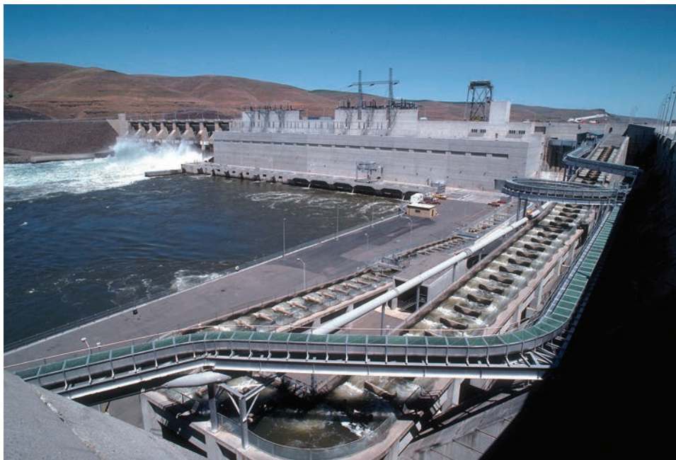
Figure 12. Given the likelihood that hydroelectric energy generation facilities will remain the only large-scale sustainable energy source in the Pacific Northwest, greatly increased efforts must be directed at resolving upstream and downstream passage for juvenile and adult salmon. (Source: U.S. Army Corps of Engineers.)
