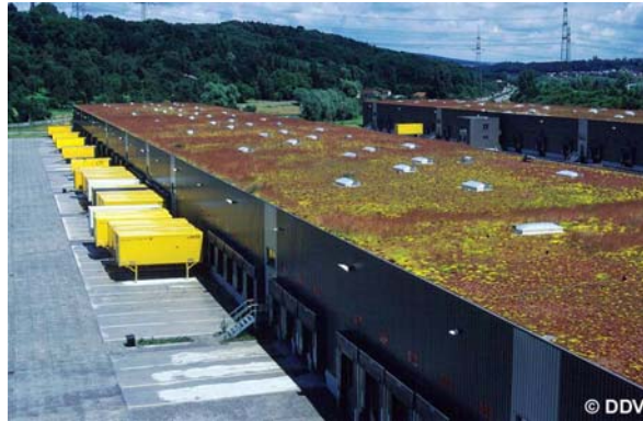
Figure 1: "Freight distribution centre" near Stuttgart, Germany.
