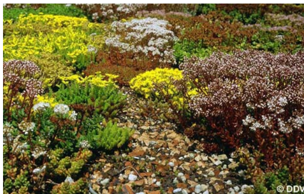
Figure 2: Green roof substrate made of recycled clay tiles
