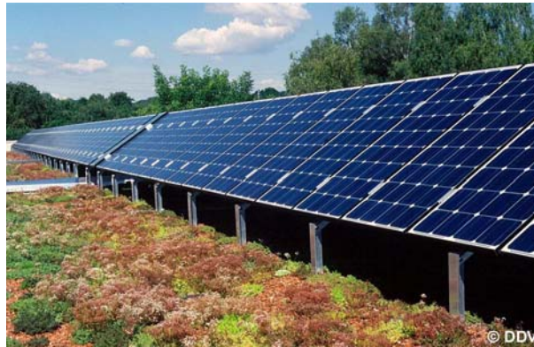
Figure 4: Photovoltaic installation combined with extensive green roof on a school near Stuttgart
