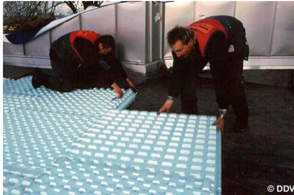
Figure 5: These elements are draining and thermally insulating at the same time
