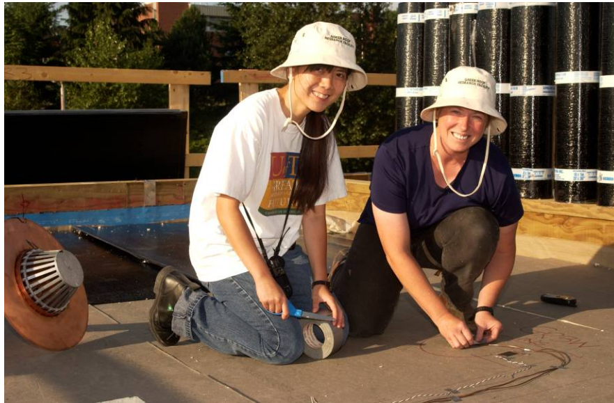
Photo 13 BCIT Green Roof Research Facility. Researchers interface temperature and heat flow sensors in the roof system.
