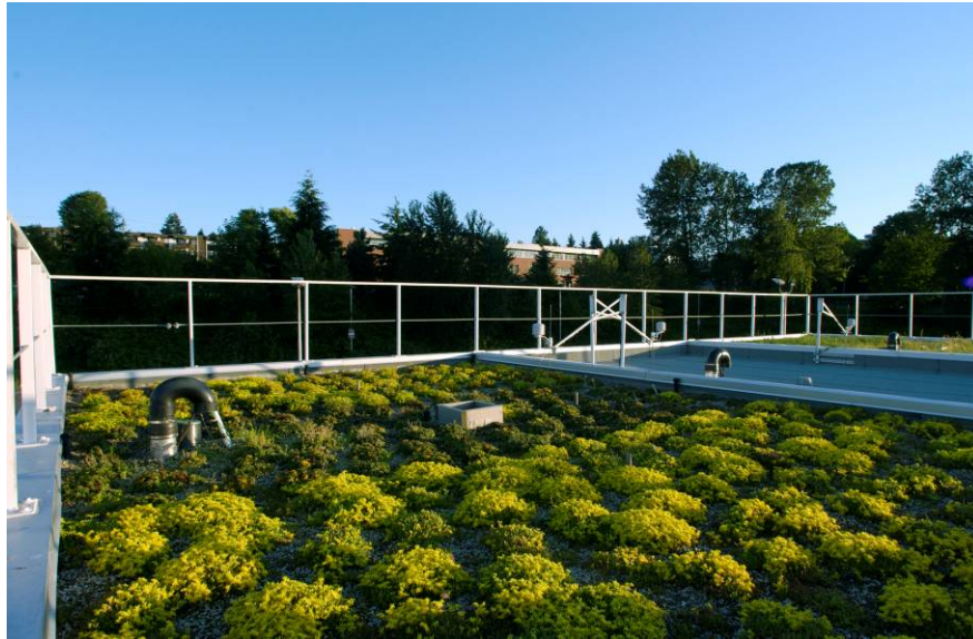
Photo 1 BCIT Green Roof Research Facility rooftop, Great Northern Way Campus, Vancouver, British Columbia.
