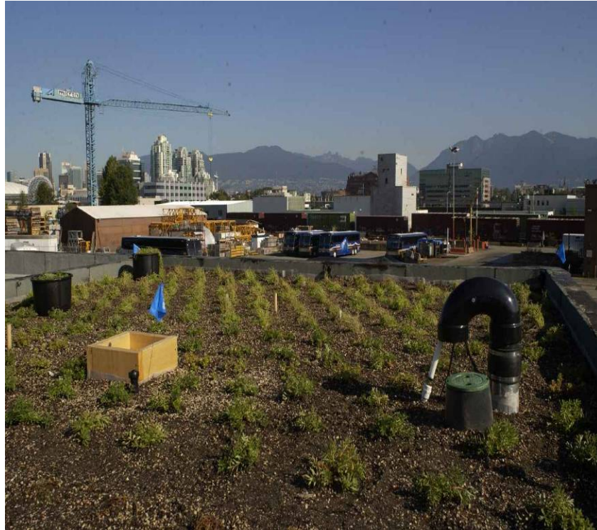
Photo 7 BCIT Green Roof Research Facility, completion of planting, summer 2003.
