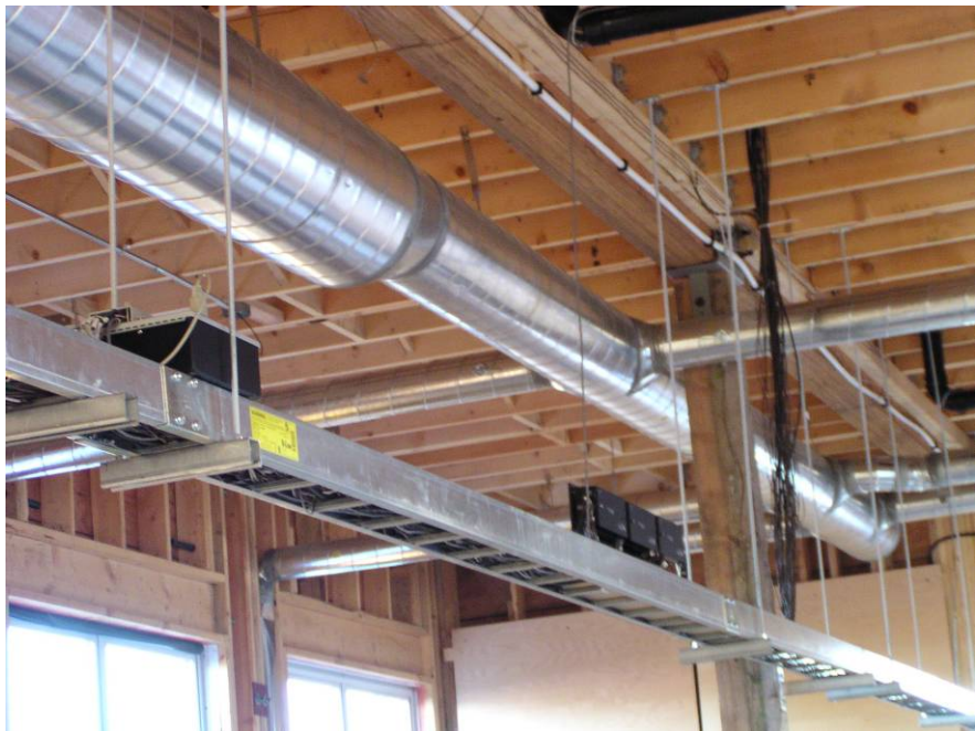
Photo 17 BCIT Green Roof Research Facility data acquisition system.
