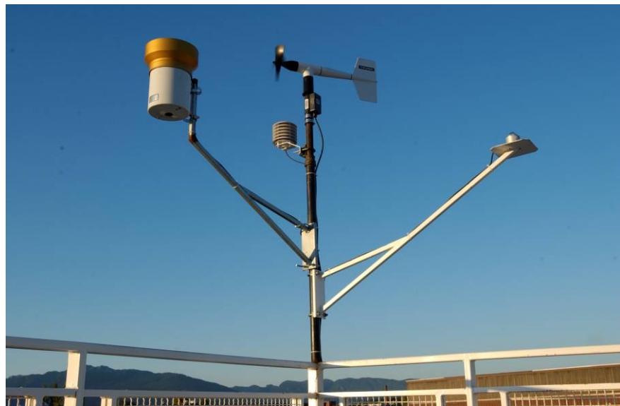
Photo 16 BCIT Green Roof Research Facility rooftop weather station.
