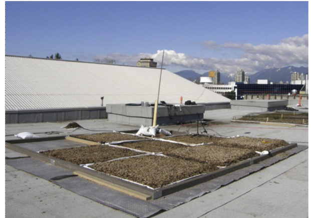
Fig. 3. Rooftop test plots of substrates with P3 community (cultivated grasses) in foreground and P1 community (sedums) in mid-ground.
