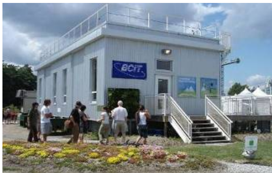
Photo 1 - Green Roof Research Facility
