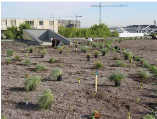
Stantec green roof in Edmonton. Photo courtesy of Stantec
