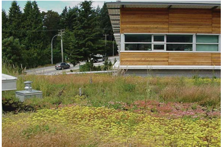
The Sechelt green roof in July 2004.
