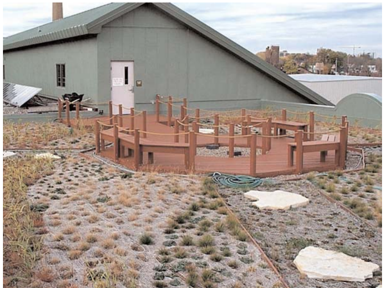
The new green roof at Minneapolis' Green Institute.
