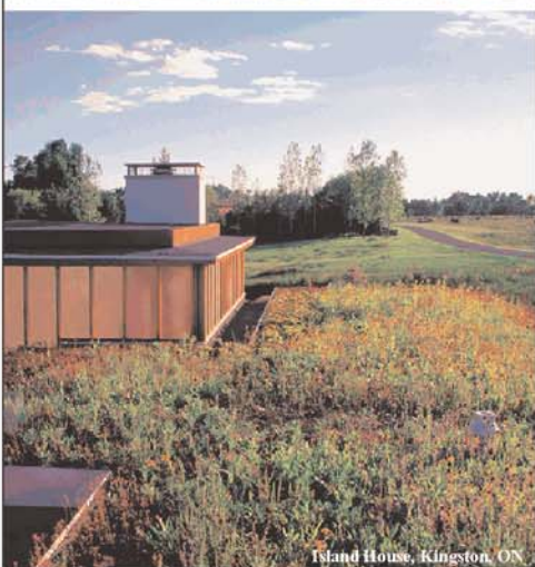
Island House, Kingston, ON
