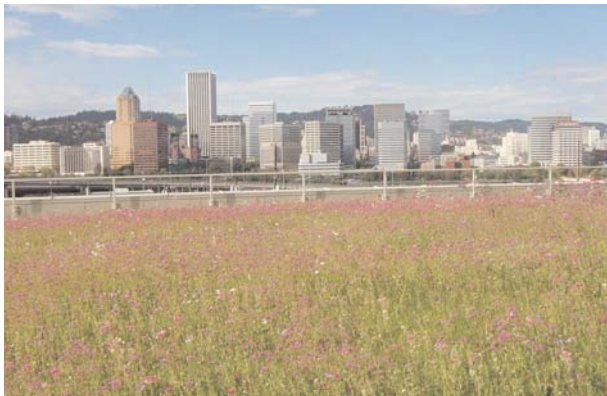
The Multnomah County Building's green roof demonstration project.
