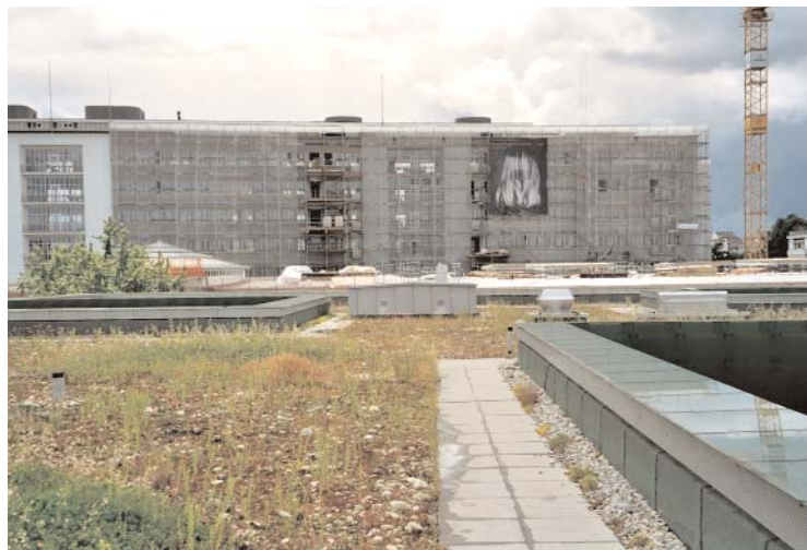
The green roof on the Kanton hospital in Switzerland. This project serves as one of the research sites for the biodiversity research being conducted by Dr. Stephan Brenneisen, whose research has shown that green roofs provide habitat for birds and invertebrates in urban areas.
